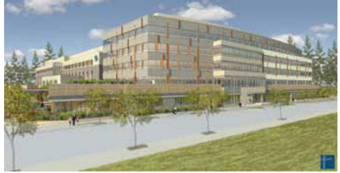
When complete, the new medical office building at Swedish/Issaquah will be home to a 15,000-square-foot comprehensive cancer care center that will offer integrated medical oncology, infusion therapy and radiation oncology services, as well as educational and support programs. Rendering courtesy of CollinsWoerman.
